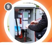
Splice the fibre bare end and connect Emtelle HomeConnect at the access chamber or cabinet.
