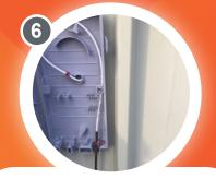
At CCE, secure 3mm LFH & 5mm PE cables as shown.
