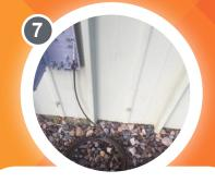
Run the cable to the nearest splice or fibre connectivity point.
