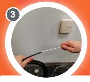
Slide and adjust the external sheath to expose LFH tube to required length.
