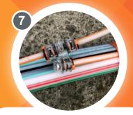
An end cap is used on the microduct once the fibre has been removed.
