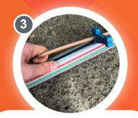
Once the blade is set, position the cutter where the cut is needed. Rotate 2-3 times, enough to score the microduct.
