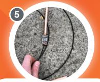
Ensure a connector is push fitted onto the end of the customer drop microduct and insert the fibre through the connector and into the microduct.
