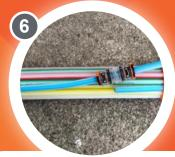
Once all the fibre has been pushed through, the customer drop microduct and connector can be push fitted onto the microduct from the bundle.
