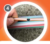
Snap the microduct on the score mark made. Pull out the required amount of fibre.
