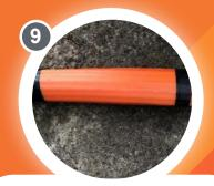
The sheath that was removed from the microduct bundle can now be taped into place, adding additional protection.
