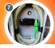
Plug in the QWKlink at the customer connection. Storing excess fibre of up to 30m.
