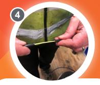
Ring cut the micro duct, remove the excess fibre and store at the customer connection point.
