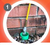
Push the duct rod from the customer connection to the main splice location, this is the best direction when using QWKConnect in a ducted network.
