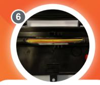
Seal the microducts and put in place within the EMU Closure.
