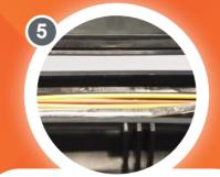
Seal off the RTRYVA appropriately and push the RTRYVA into place within the EMU Closure.
