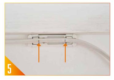
Place the cable within the Break-Out Bend Manager and mark start and end points for a window cut.
