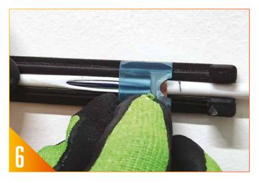
Remove from the Break-Out Bend Manager and use a window cutting tool to access the fibres.
