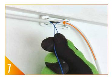
Place the cable back into the Break-Out Bend Manager, now the fibre can be selected and pulled back.
