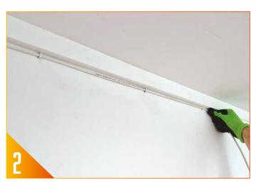
Drill the required holes for all FireClips and push clips over the RTRYVA cable to fix into place.
