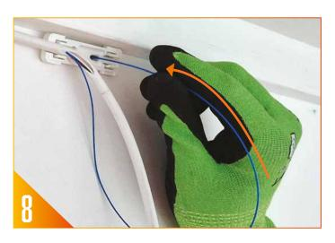
Once the fibre has been retracted, start pushing it through the drop tube to the other side of the wall into another Break-Out Bend Manager.
