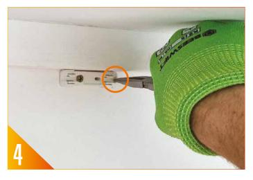
Place and fix to the wall with a screw and if the cable is continuing its route for more fibre drops, remove the end cap to allow the cable to pass through.
