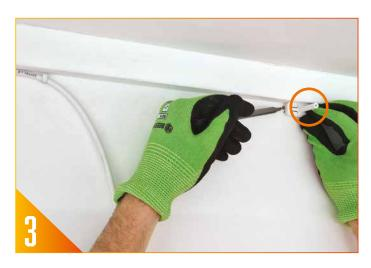
Using the Break-Out Bend Manager, mark out and drill the passage for the fibre drop to the other side of the wall.
