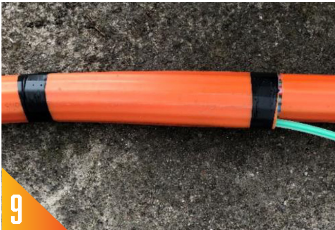
9 The sheath that was removed from the microduct bundle can now be taped into place, adding additional protection.
