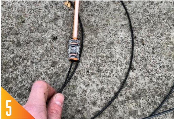
5 Ensure a connector is push fitted onto the end of the customer drop microduct and insert the fibre through the connector and into the microduct.
