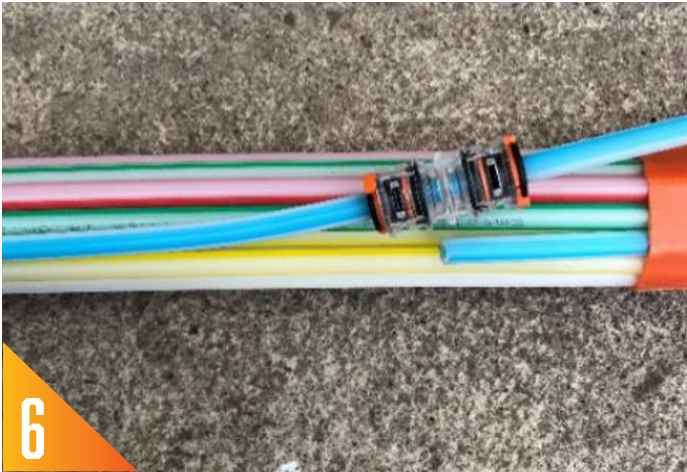
6 Once all the fibre has been pushed through, the customer drop microduct and connector can be push fitted onto the microduct from the bundle.
