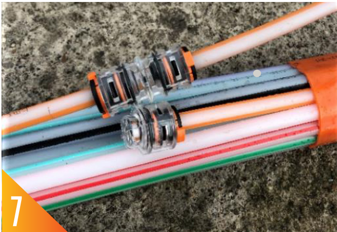
7 An end cap is used on the microduct once the fibre has been removed.
