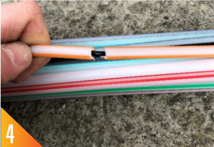
4 Snap the microduct on the score mark made. Pull out the required amount of fibre.
