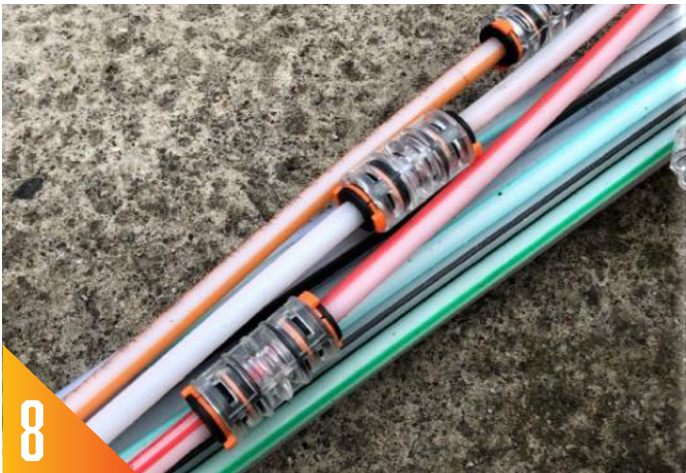
8 If two or more customer connection drops are needed, the straight connectors have to be staggered along the length of the longitudinal cut.
