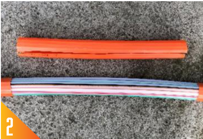
2 Remove the sheath but do not throw away. The selection of microduct can now be made.
