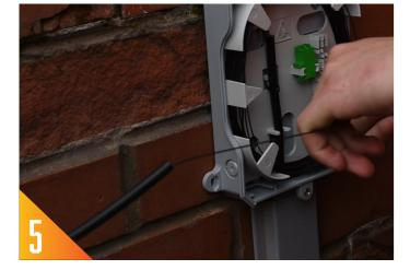
After securing the microduct into the enclosure – slowly retrieve the FibreFast Microcable while neatly storing into the enclosure slack storage tray.
