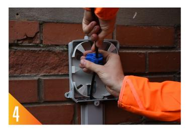
Measure the microduct requirement length and carefully ring cut the excess microduct away from the FibreFast Microcable.
