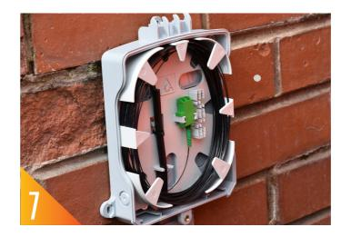
The optical connector can now be plugged into the customer termination enclosure.
