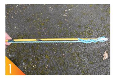
Push the duct rod from the customer termination point to the main distribution node pulling in a rope, this is the best direction when using QWKconnect in a ducted network.
