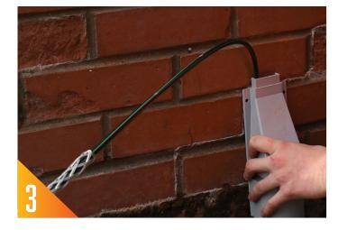
Pull all the excess QWKconnect through to the customer termination point. Neatly managing the duct slack.
