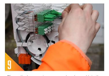
The optical connector can now be plugged into the distribution node completing the full installation.
