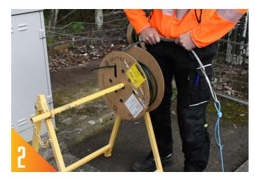
Attach the pulling rope with a fuse and pulling sock onto the QWKconnect and pullback through to the customer termination point.
