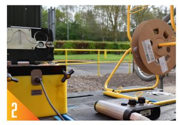
Securely mount the cardboard reel onto a cable drum stand. Ensure the stand is aligned with the blowing machine with no sharp bends.
