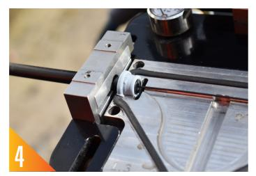
Feed the cable by hand through the blowing machine into the receiving microduct, about 10m. Ensure the QWKlink can freely move inside the machine and microduct.
