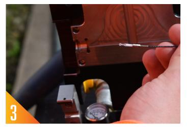
Remove the outer QWKlink cable end with the blowable ferrule and proceed to insert the QWKlink into the blowing machine. Ensure the dust cap is present.
