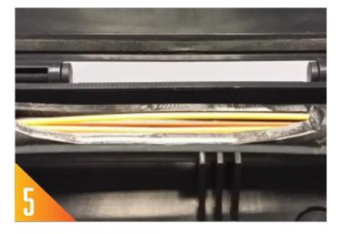
Seal off the RTRYVA appropriately and push the RTRYVA into place within the EMU Closure.
