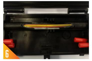
Seal the microducts and put in place within the EMU Closure.
