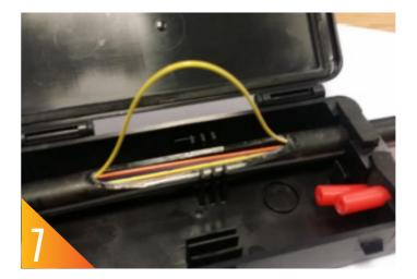
The fibres can now be selected to be pushed or pulled back to the desired drop microduct.
