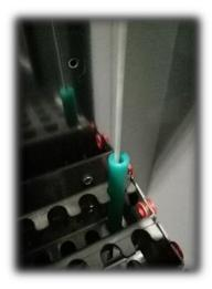
Locate the microduct and identify the fibre unit that needs restrained, select the correct ELF.
