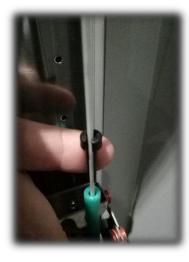
Starting with the front of the ELF (closest to microduct) gently push the fibre into the central channel until the fibre is secure.
