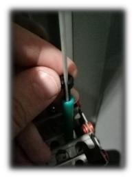
Using the top of the ELF push it into the microduct to activate.
