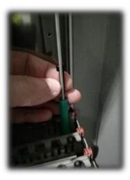
Line up the ELF central channel with the fibre unit.
