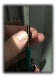
Line up the ELF central channel with the fibre unit and push the fibre into the slot.
