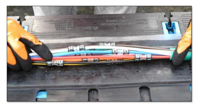
**Step 3**Begin to wrap the EM-WRAP around the duct/tube assembly.
